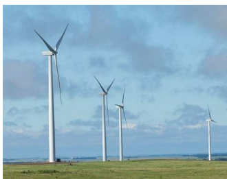
Images courtesy of Basin Electric Power Company
